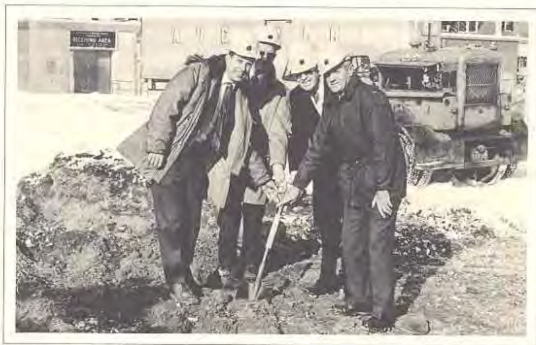
Groundbreaking. Dr. McIntyre (left) and Senator Cotton (second from right) don hard hats for the occasion.
